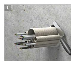
Choose the pipe collar according to the single pipe or bundle. The inner diameter of the pipe collar should not be bigger than 30 mm than the single pipe or bundle.
