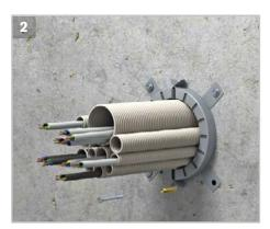
Strap the single electrical lines to bundles by using an adhesive tape. Fill remaining spaces of the wall or floor with mortar or gyp-
