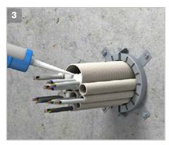
Fix the pipe collar by the appropriate rawlplugs and screws or threaded rods, respectively. For wall installations one pipe collar on each side of the wall and for floor installations one collar on the underside of the floor must be provided.
